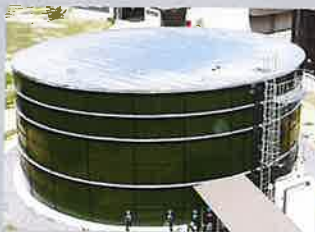
Trough Deck Roof
