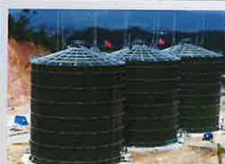
Tapered Steel Roof
