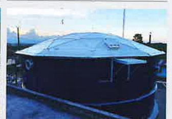
Geodesic Dome Roof
